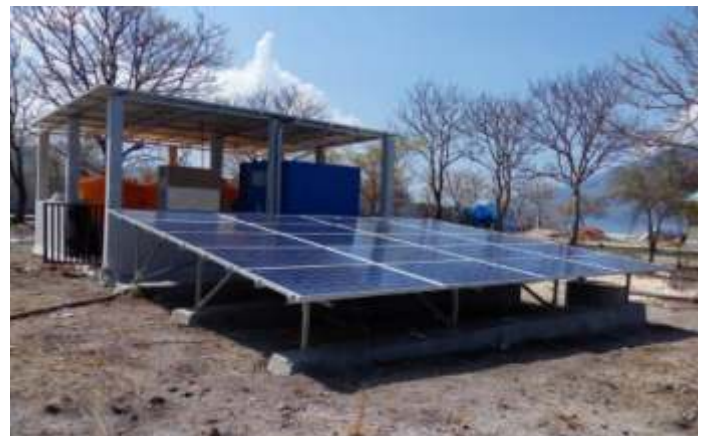
SWRO With Solar Cell Cap. 9000 L/Day, Installed more than 200 units in Indonesia
